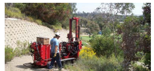
Limited Access Drilling
