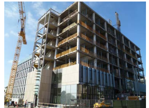
University of California San Diego Biomedical Research Facility Unit II
